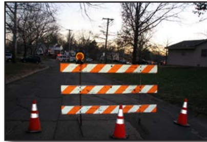
Figure 8.24 – In some cases, a street may need to be closed for an extended period. (Photo/Mike Wieder)
