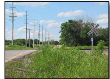
Figure 7.7 – Consider an unguarded railroad crossing sign and a signal to stop. (Photo/Mike Wieder)
