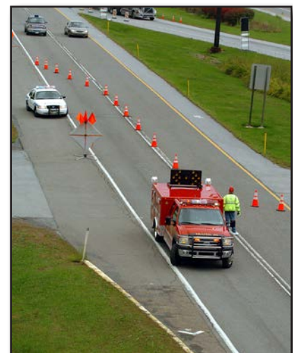
Figure 7.4 – The advanced warning area provides a measure of security for the incident work area. (Photo/Bob Esposito, Pennsburg, Pennsylvania)
