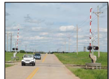
Figure 7.8 – Use caution when approaching any railroad crossing, with or without crossing gates. (Photo/Mike Wieder)
