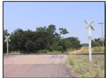
Figure 7.13 – A typical unguarded rail crossing, often found in rural areas. (Photo/Mike Wieder)
