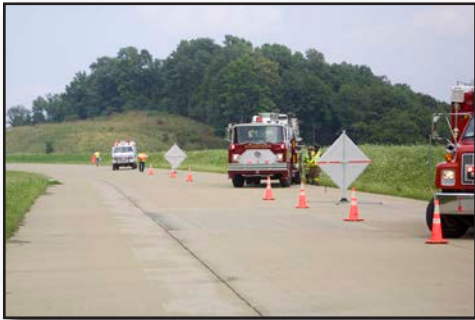
Figure 7.35 – The flagger should be in the lane adjacent to flowing traffic. (Photo/Bob Esposito, Pennsburg, Pennsylvania)
