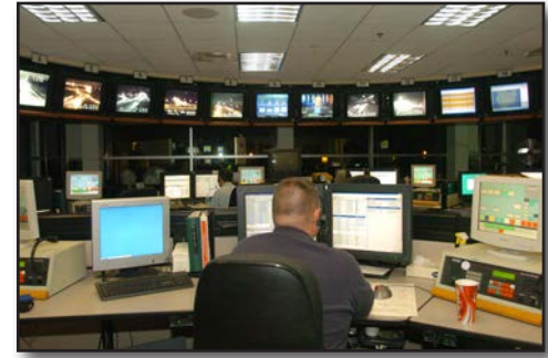
Figure 6.1 – Traffic control centers have myriad equipment used to monitor traffic and road conditions. (Photo/Bob Esposito, Pennsburg, Pennsylvania)
