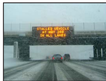
Figure 6.4 – Changeable message signs alert motorists to hazardous road conditions.
