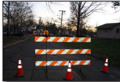
Figure 8.24 – In some cases, a street may need to be closed for an extended period. (Photo/Mike Wieder)
