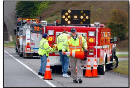
Figure 7.2 – Use extreme care when placing traffic control devices on an active roadway. (Photo/Bob Esposito, Pennsburg, Pennsylvania)
