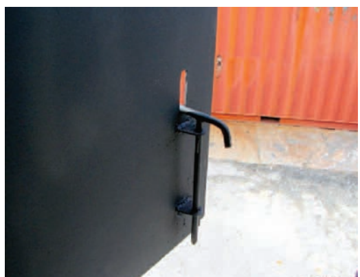
Figure C-6: Window & Latch Construction
