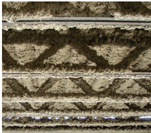
Figure C-4: Fireproofing added to structural steel
