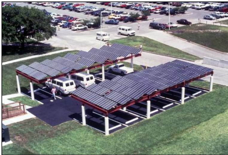
Figure 5-9: An EV Fleet Charging Station (Photo courtesy of NREL Photographic Information Exchange)
