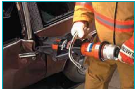
spreading a door from the vehicle
