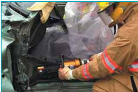
dash lift using combi-tool
