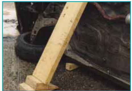
wood type shoring
