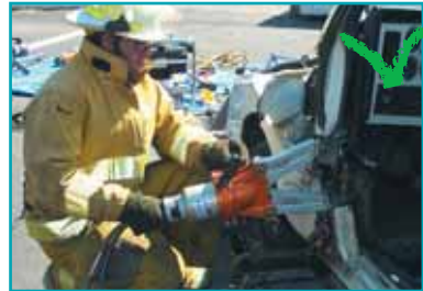
correct spreader positioning
